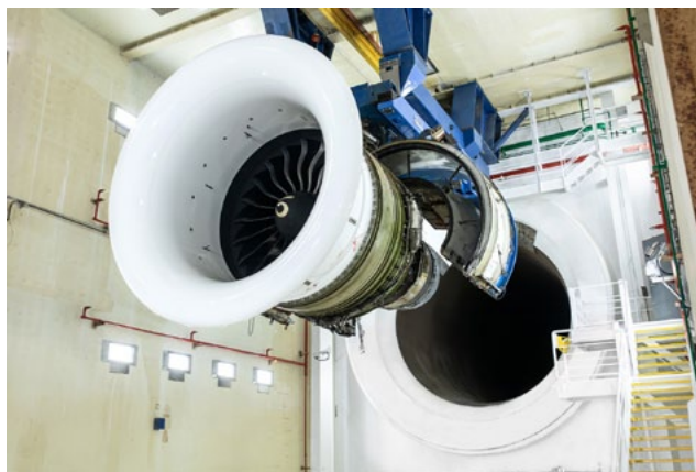
To prepare for the future entry of the GE9X series engine into the market, HAECO commenced a major modification of its engine test cell Photo: HAECO
